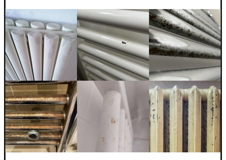
The images above show issues such as rusting, peeling, discoloration, and tarnishing, all resulting from improper cleaning of radiators and towel rails.
